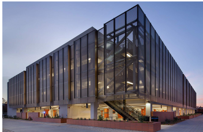
THE PERFORATED METAL PANEL SCREEN SYSTEM AT STANFORD UNIVERSITY PARKING GARAGE. PHOTO BY BERNARD ANDRE.
