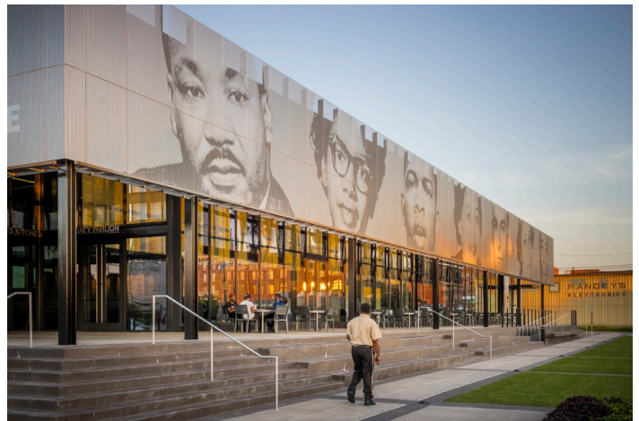
ZAHNER IMAGEWALL WAS USED TO CREATE THE CUSTOM PERFORATED FACADE THAT CLADS THE AWNING OF THE EJI LEGACY PAVILION. PHOTO BY CORNELIUS HAYES, ARKO | © A. ZAHNER COMPANY
