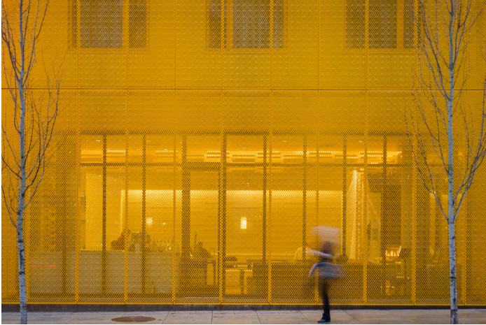
EXTERNAL PRIVACY AND SHADING SCREEN FOR THE RESIDENCE INN. ROUND EMBOSMENT PUNCHES IN PANELS ADD RIGIDITY IN ADDITION TO VISUAL TEXTURE. PHOTOS © BEN COFFMAN.
